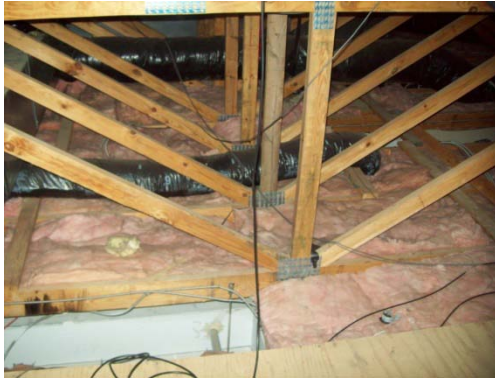
Attic insulation with bays missing insulation
