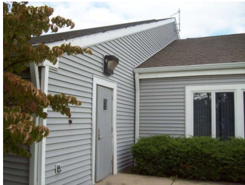
Typical Exterior wall of building
