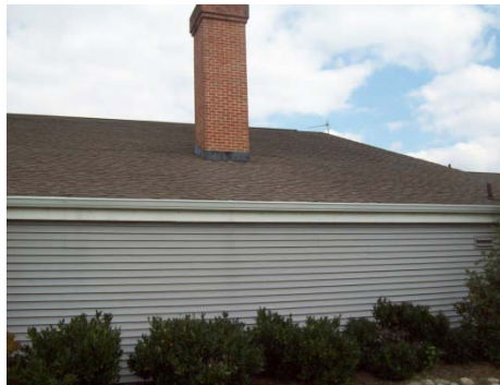
Asphalt shingle roof
