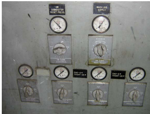
Pneumatic Control System Panel in C/D Wing Boiler Room
