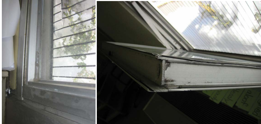
Single pane aluminum framed windows
