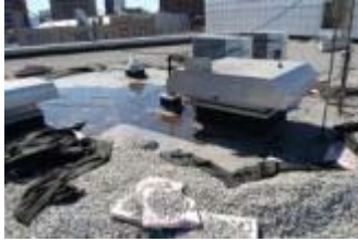
Signs of standing water/pooling
