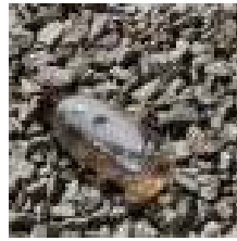
Rocks/nails or other sharp objects on roof surface
