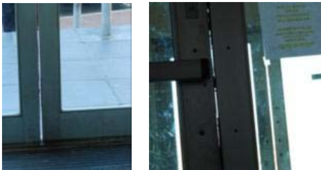
Missing/worn weather-stripping
