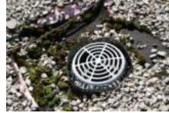
Clogged/damaged roof drains
