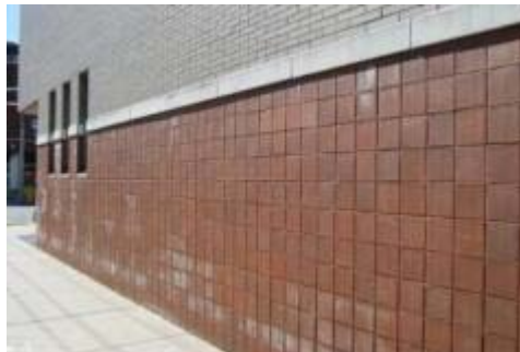
Efflorescence on brick and masonry walls indicate moisture presence within the wall cavity.
