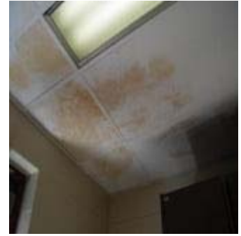
Signs of mold/water damage on interior ceiling tiles
