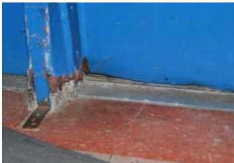
Damaged and aged door frame
