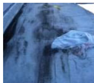
Signs of standing water/pooling
