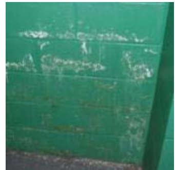
Efflorescence on brick and masonry walls indicate moisture presence within the wall cavity.
