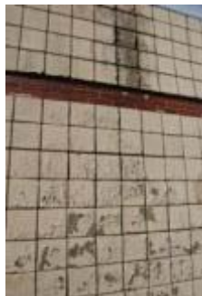
Signs of uncontrolled roof water runoff on walls due to missing/defective roof flashing
