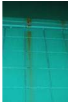
Signs of roof leakage on interior wall surfaces.
