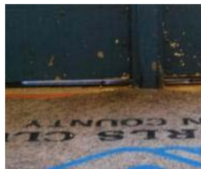
Missing/worn weather-stripping
