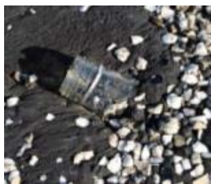
Broken glass and other sharp objects on roof surface
