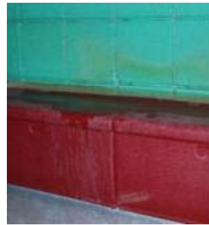
Signs of extensive roof leakage on interior equipment and finishes throughout the building, especially in the gymnasium
