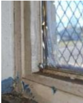
Damaged/aged window frame
