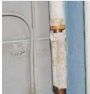
Signs of extensive roof leakage on interior equipment and finishes throughout the building, especially in the gymnasium
