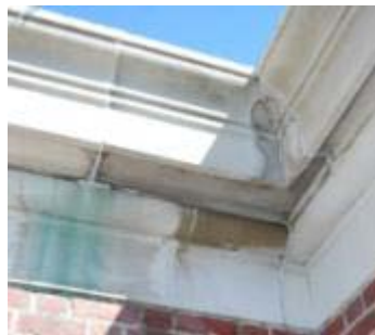
Signs of uncontrolled roof water runoff on walls due to missing/defective roof flashing
