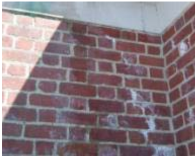
Efflorescence on brick and masonry walls indicate moisture presence within the wall cavity.
