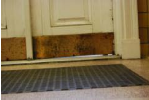
Missing and worn weather-stripping found
