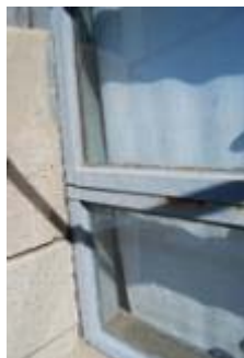
Single-glazed window with ineffective frame
