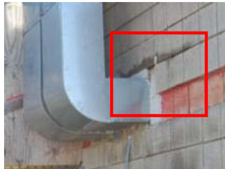
Signs of water damage at perimeter walls
