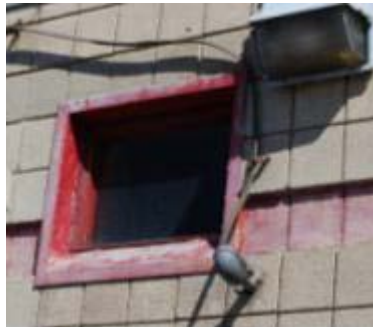
Single-glazed window with ineffective frame
