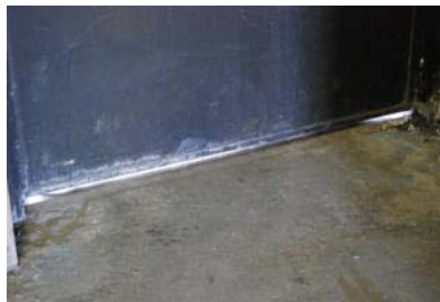
Missing/worn weather-stripping
