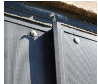
Warped/aged metal door frame
