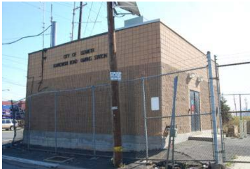
Front and Left Side Façade
