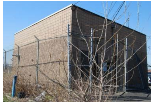
Rear and Right Side Façade
