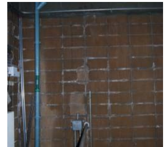
Deteriorating exterior and interior wall finishes due to water and moisture presence inside the wall cavity
