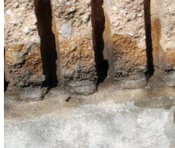
Deteriorating exterior and interior wall finishes due to water and moisture presence inside the wall cavity
