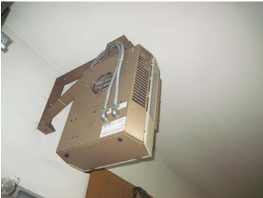
Existing Electric Heater
