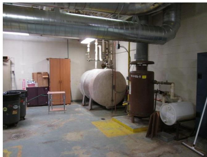
3: Existing Domestic Hot Water Heater
