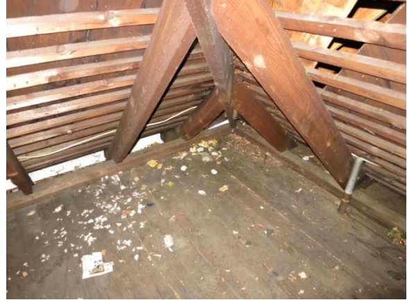
Image 3: Sample Attic Flooring and Roof Condition
