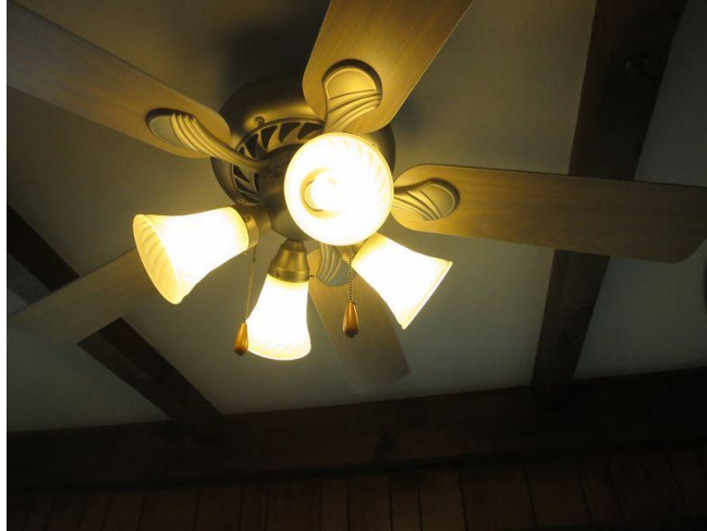
Image 10: Compact Fluorescent Fixture in Front Office Area
