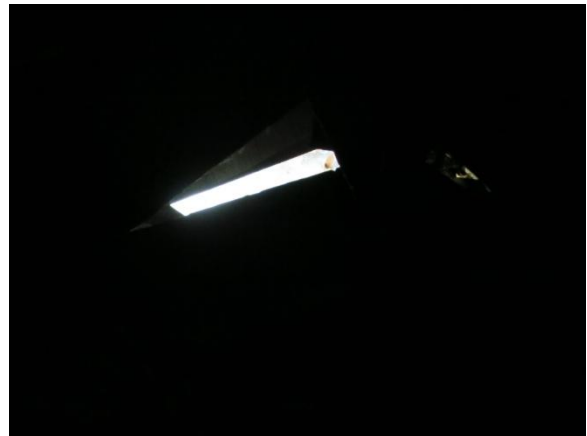
Image 5: Sample of Roof Opening
