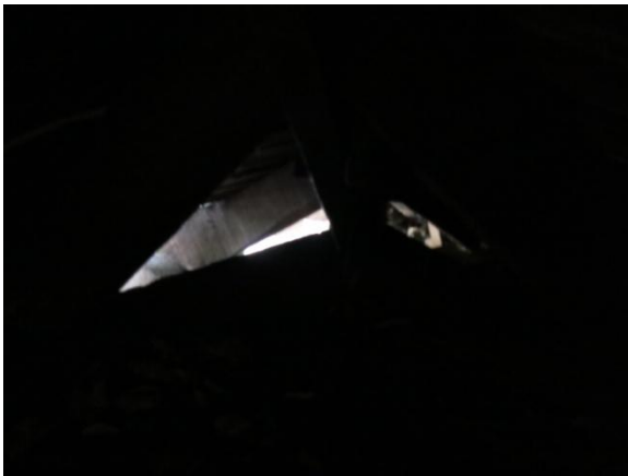
Image 4: Sample of Roof Opening
