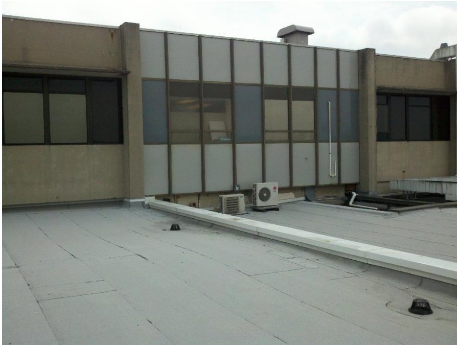
1. Second story windows to be replaced
