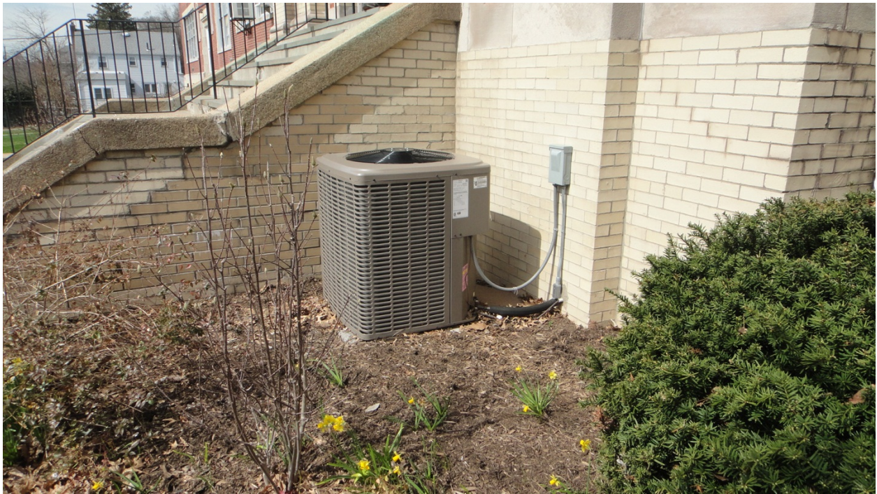
AIR COOLED HEAT PUMP CONDENSING UNIT SERVING KINDERGARTEN
