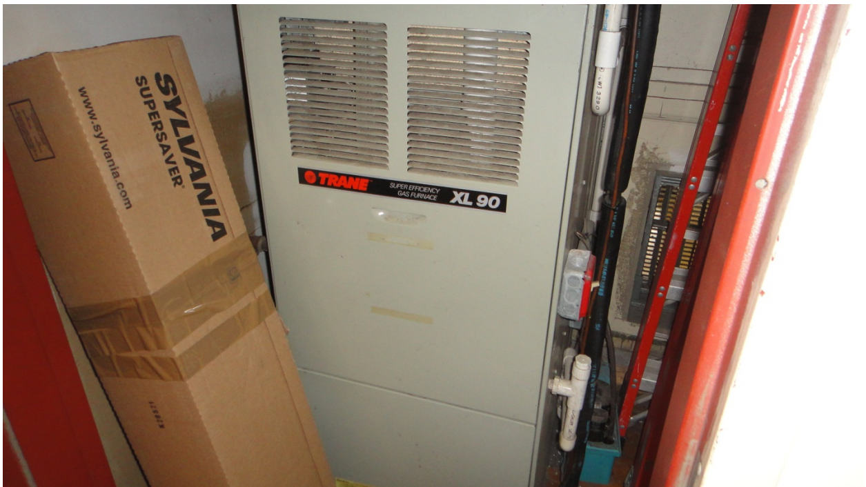
INDOOR UNIT OF DX SPLIT UNIT SERVING SECOND FLOOR CLASSROOM
