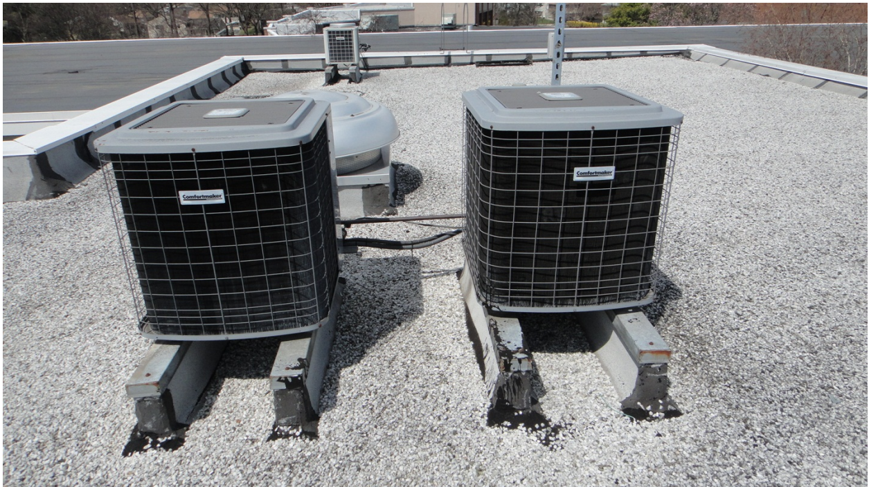
AIR COOLED CONDENSING UNITS SERVING HALLWAYS OF NEW WING
