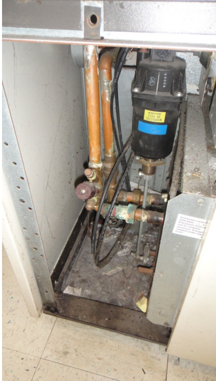
INTERIOR OF UNIT VENTILATOR
