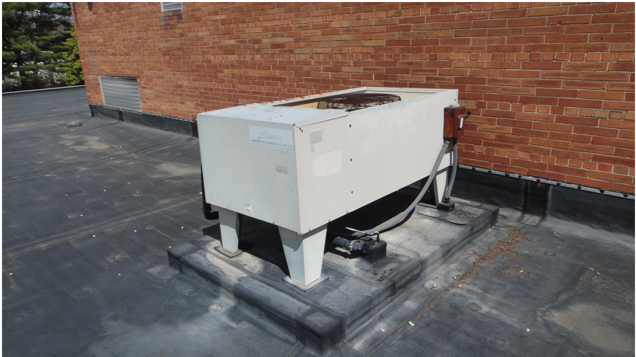
AIR COOLED CONDENSING UNIT SERVING OFFICE AREAS
