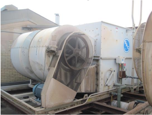
Existing Cooling Tower
