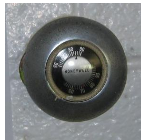
Dorchester ES Unit Ventilator Pneumatic Thermostat
