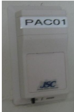
Woodcliff MS Room 21 thermostat with slider to the left on full cold
