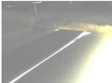
Open seams in lighting fixture
