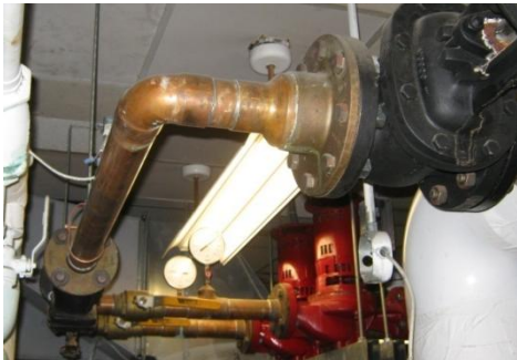
Dorchester ES bare heating hot water piping
