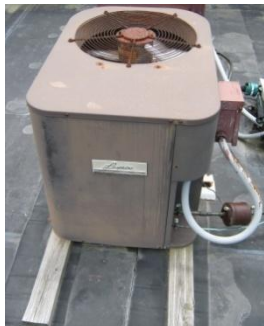
DX condensing units located on the roof at Woodcliff Middle School
