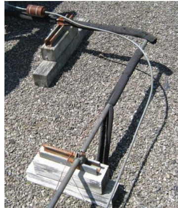
Dorchester ES refrigerant piping with missing insulation
