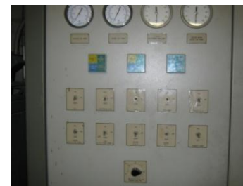
Dorchester ES unit ventilator time clock. Pins are not set.
