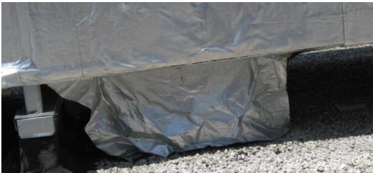
Woodcliff MS Cafeteria RTU damaged insulation
