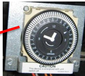
Dorchester ES unit ventilator time clock. Pins are not set.
