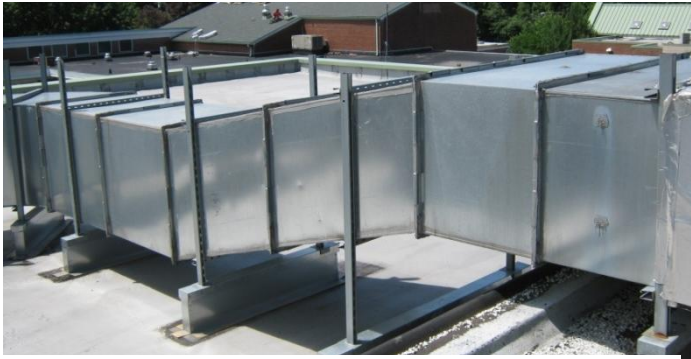
Woodcliff MS Cafeteria RTU bare ductwork
