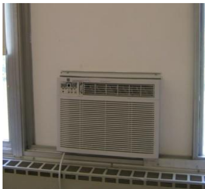
Window AC unit at Dorchester Elementary installed in uninsulated panel
