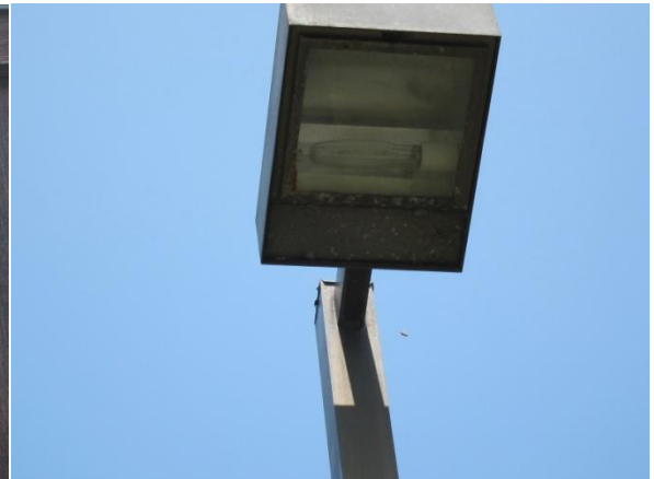
Wall Mounted Metal Halide Exterior and Parking lot lights
