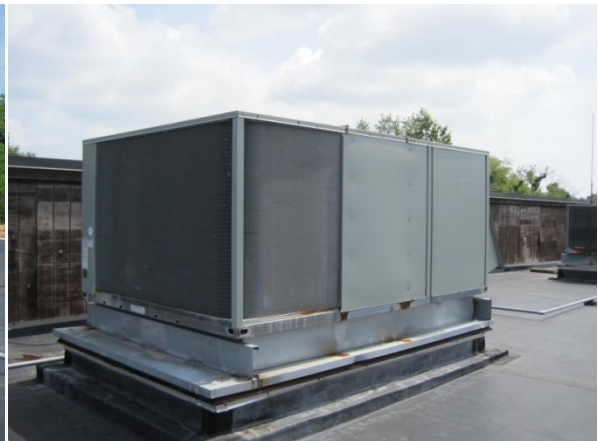
The multipurpose/Court room unit
