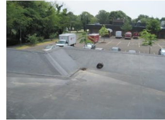
Cap removed from drainage pipe
