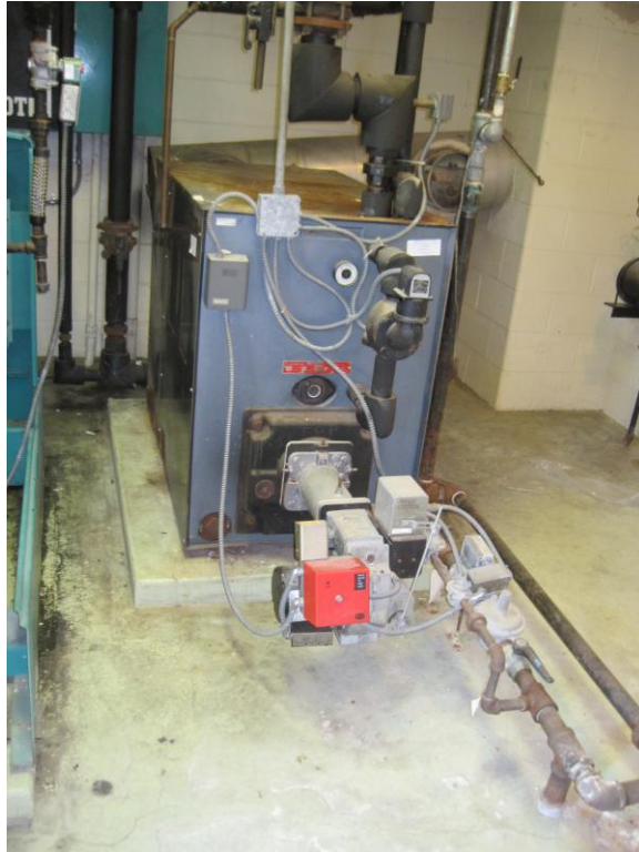
The Weil-McLain 480MBtu/hr cast iron sectional boiler
