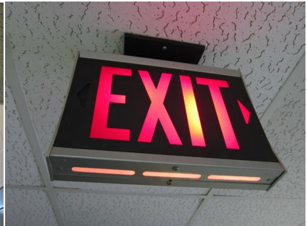
Typical incandescent Exit Signs seen throughout the building
