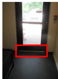
Missing/worn weather-stripping
