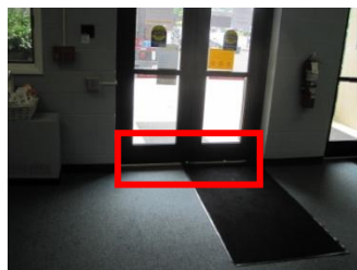
Missing/worn weather-stripping
