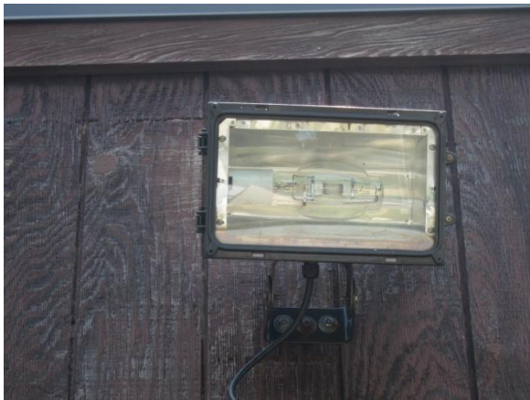
Wall Mounted Metal Halide Exterior and Parking lot lights
