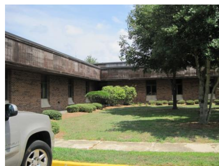
Southwest Facing Façade
