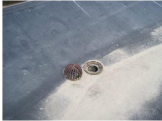
Cap removed from drainage pipe
