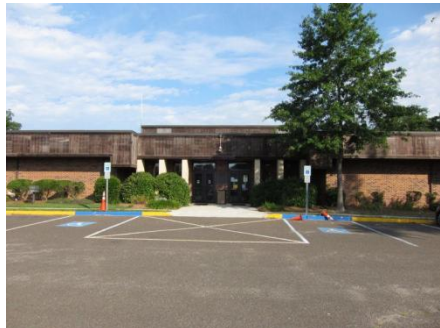
Southeast Façade and Main Entrance
