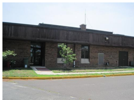
Northwest Façade and Rear Entrance
