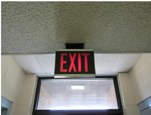
Typical incandescent Exit Signs seen throughout the building
