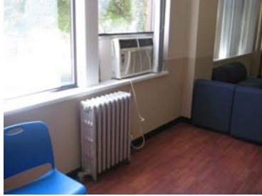
Steam radiator on ground floor
