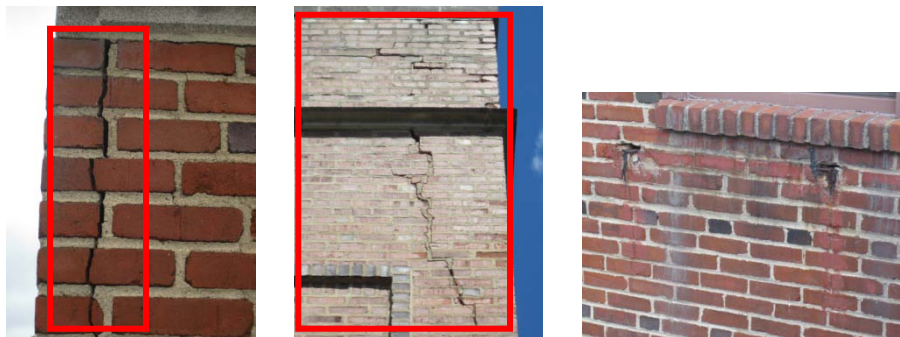
Cracked/deteriorated bricks and mortar joints
