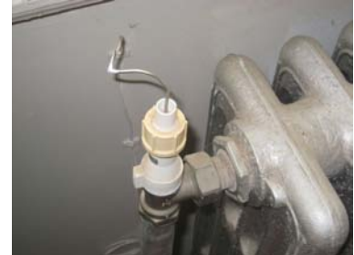
Manual valve on steam radiator
