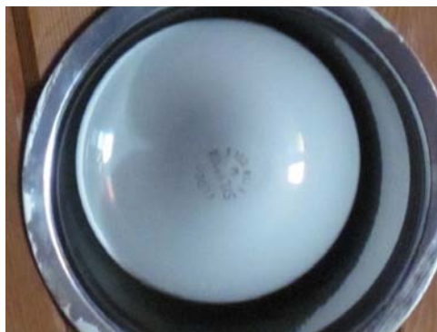
100W incandescent flood lamp found in recessed fixture in Theater
