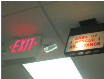
LED exit sign next to incandescent Area of Rescue sign
