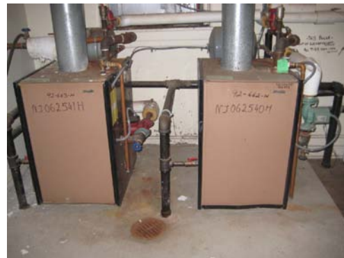
3 rd and 4 th floor hot water boilers
