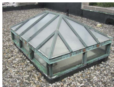
Single pane glass skylight over 4 th floor – in need of repair/caulking
