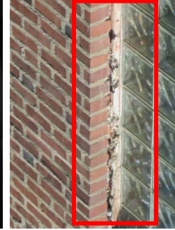
Cracked or aged caulk around frame/sill on the exterior
