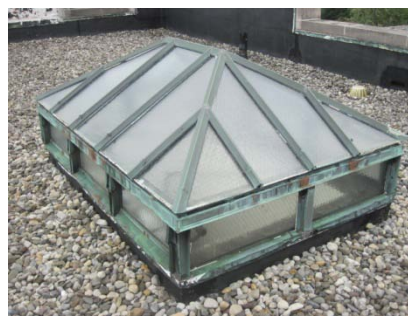
Cracked aged brittle caulk around perimeter of glass skylight
