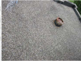
EPDM roof membrane with gravel
