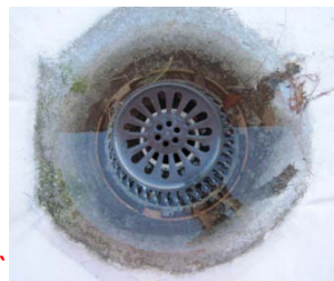
Debris filling corner of roof
