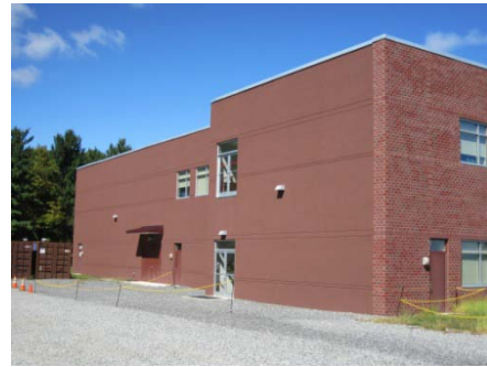
Typical building facades - EIFS and brick veneer
