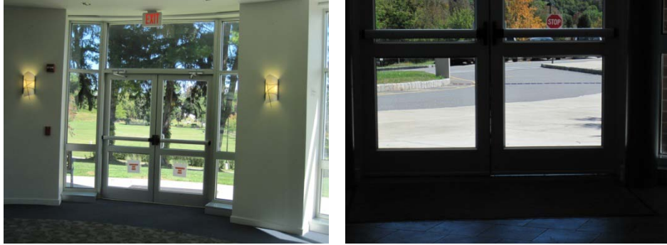
Images show typical building doors with need for regular maintenance to verify weather-stripping
