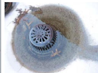
Debris clogged scupper with 2-3" standing water
