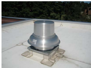
Typical Ventilation rooftop fan
