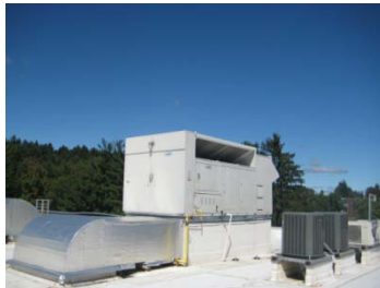
Roof top packaged unit
