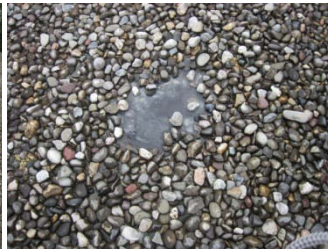
EPDM roof membrane with gravel
