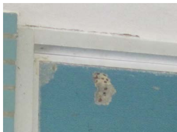
Insect burrowing in exterior wall section near main entrance
