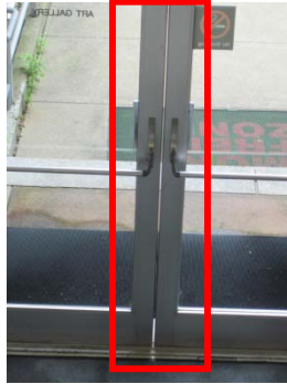
Two door types at side entrances of building in need of weather-stripping
