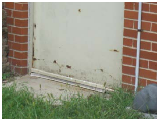
Metal rusted door at side entrance
