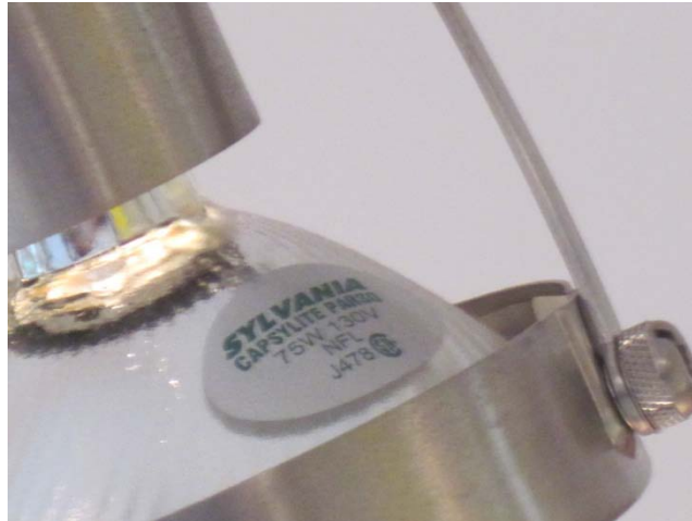
75w incandescent flood lamp found in track lighting in Gallery
