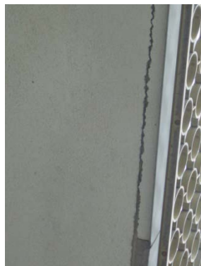
Cracked stucco in overhang ceiling at main entrance to building
