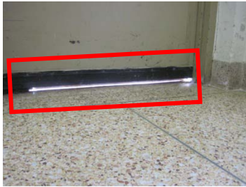
Two door types at side entrances of building in need of weather-stripping
