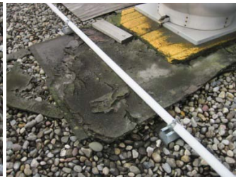
Rotted plywood under ventilation fan
