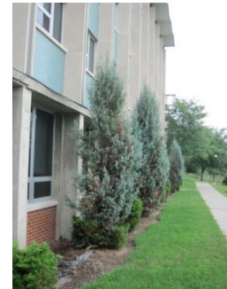
Overgrown ground vegetation touching exterior wall surfaces
