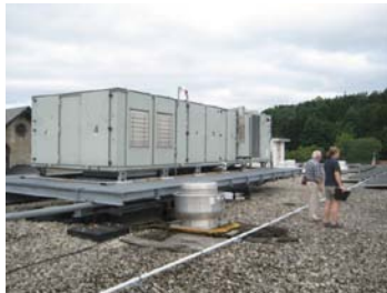
Roof top packaged unit
