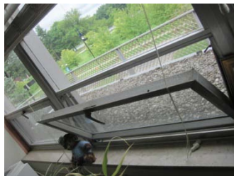
Single-glazed window with ineffective frame
