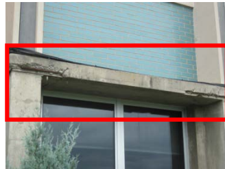
Horizontal CMU projections are directly exposed to the elements, lacking cover or flashing
