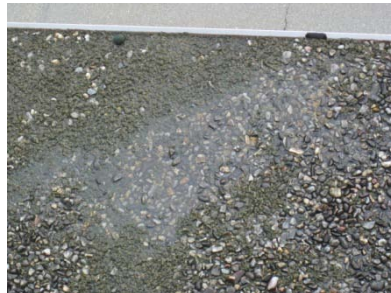
Pooled water without sufficient drainage pitch
