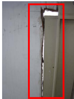
Air-leakage at sleeved window/wall air-conditioning units
