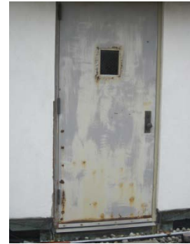
Side door showing signs of rust
