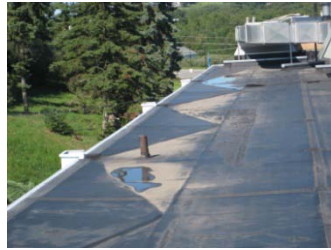
EPDM membrane, minimal standing water due to pitch
