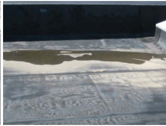
Pooling on roof
