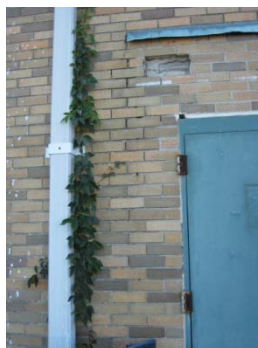
Overgrown ground vegetation touching/blocking exterior wall surfaces, missing brick veneer
