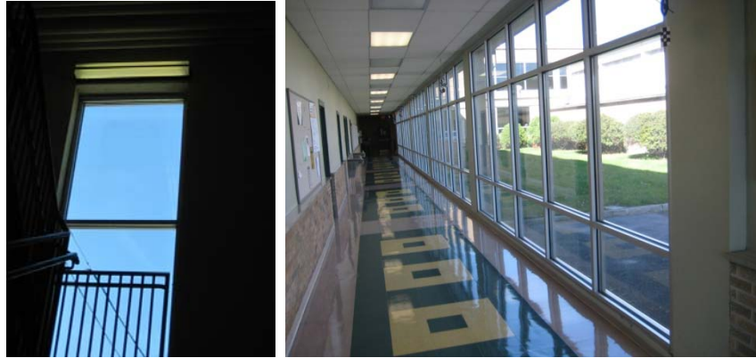
Light fixture directly over window; Hallway with sufficient daylighting without need for artificial lighting
