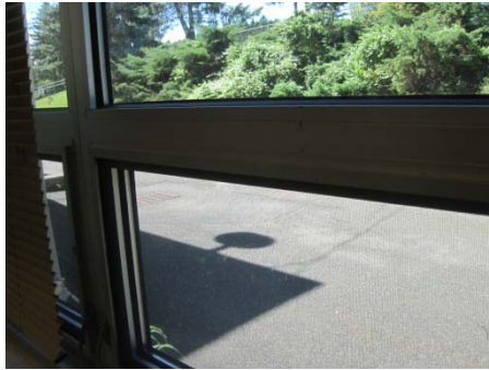
Typical aluminum frame low-e window
