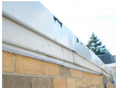
Roof tar melting around perimeter of roof
