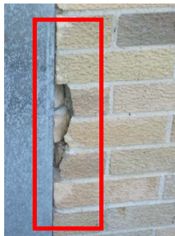
Cracked/deteriorated bricks and mortar joints
