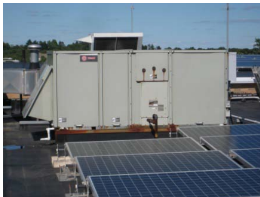
Typical Trane Roof Top Unit
