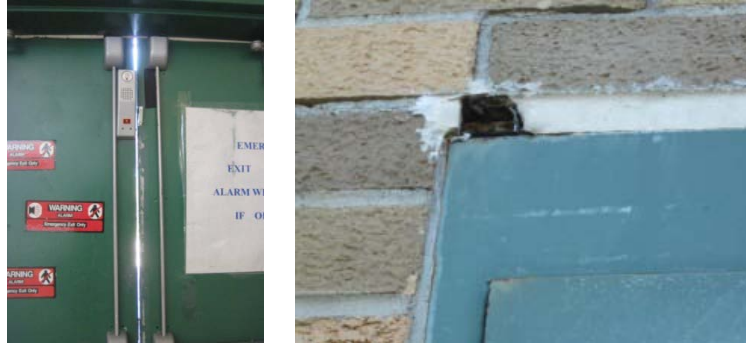
Gymnasium back doors in need of either replacement of weather-stripping and exterior caulking around perimeter of door framing
