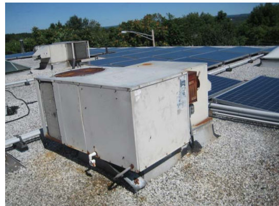
Lennox units installed in 1986: bad shape
