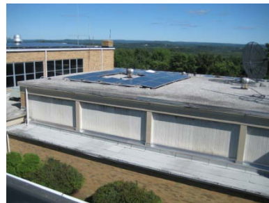
Different roofing materials – gravel built up, light colored EPDM and dark colored EPDM
