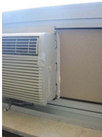
Daylight seen around perimeter of window AC unit
