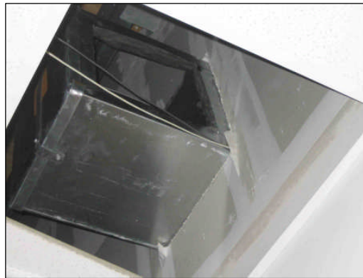
Spotswood High School – Pictures depicting exhaust/return air ending in plenum space
