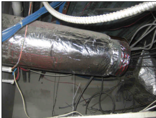
Spotswood High School – Pictures depicting exhaust/return air ending in plenum space
