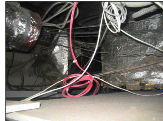
Spotswood High School – Pictures depicting exhaust/return air ending in plenum space
