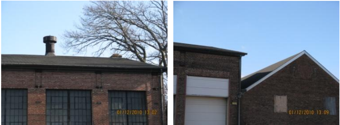
Examples of asphalt shingle roofing found throughout the entire facility
