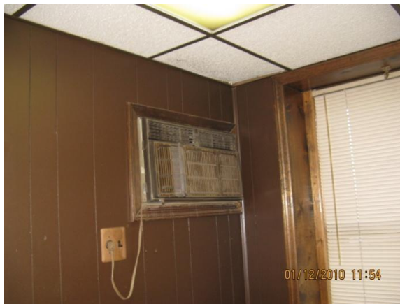
Air Conditioner Mounted In an Interior Wall
