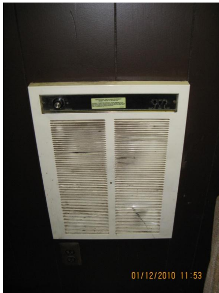
Existing Electrical Space Heaters
