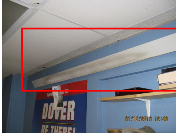
Existing Perimeter Electrical Heating
