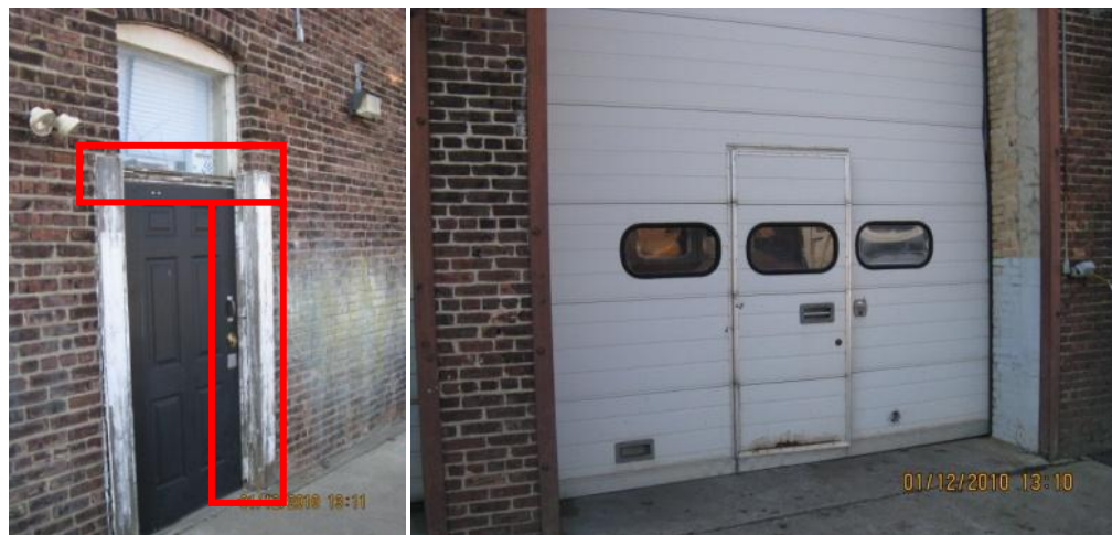
Examples of typical doors and damaged/ warped/ aged door frame, obstructed metal doors, and missing and worn weather stripping
