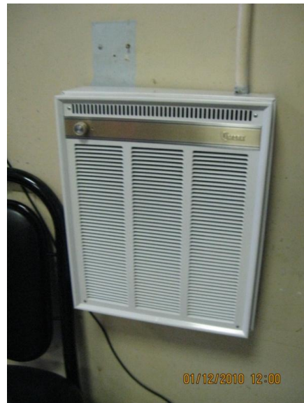
Existing Electrical Space Heaters
