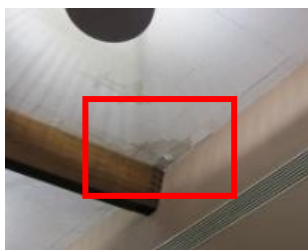
Signs of mold/water damage on interior finishes throughout the building's ceiling
