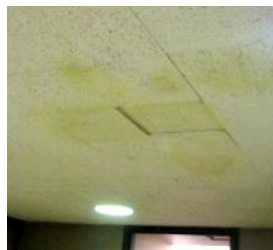
Signs of mold/water damage on interior finishes throughout the building's ceiling
