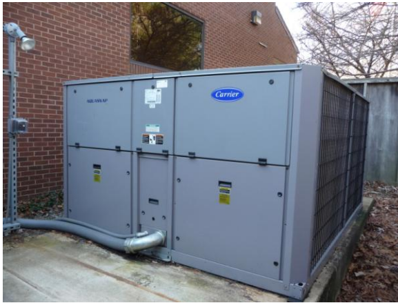
New 45 ton Carrier chiller, two views
