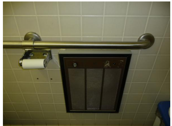
Fin-tube wall mounted hot-water radiators; small electric heaters in bathrooms - typical
