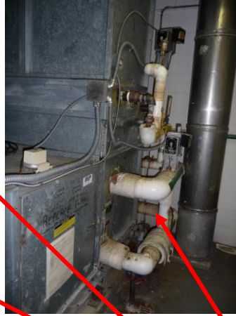
Weil McLain boiler and PowerFlame burner; AHU-1heating/cooling coils; AHU-3heating/cooling coils; thermostat
