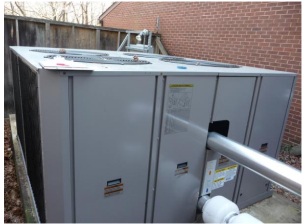
New 45 ton Carrier chiller, two views
