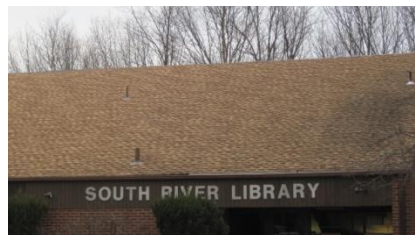
The roofing material has reached the end of its expected useful lifespan
