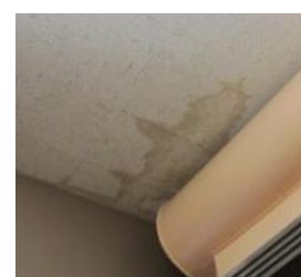
Signs of mold/water damage on interior finishes throughout the building's ceiling
