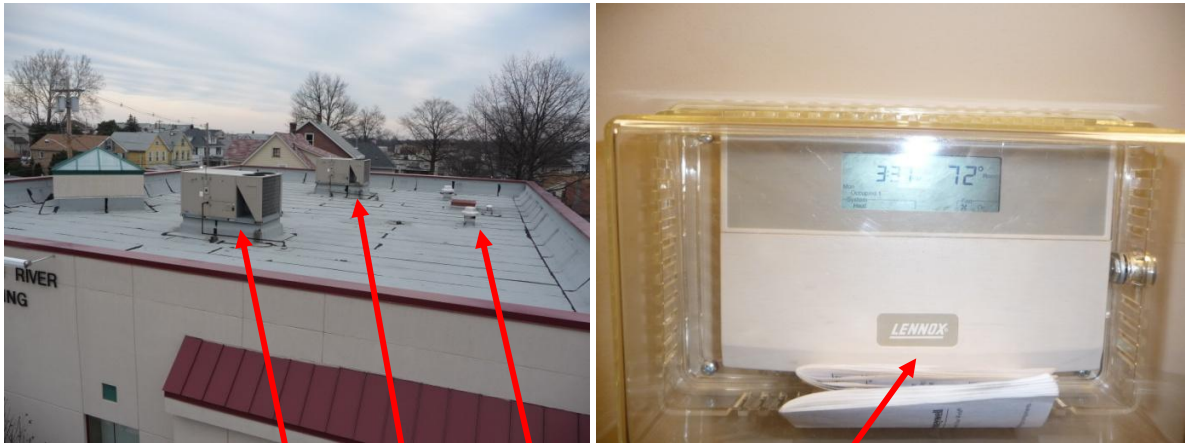
AC-2 and AC-1, 2 exhaust fans, a programmable thermostat
