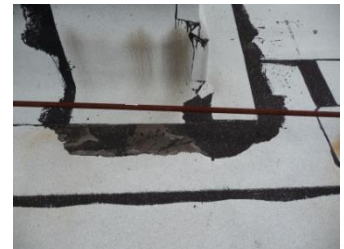
Delaminating roof membrane / patches
