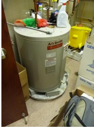
High efficiency A. O. Smith electric DHW heater
