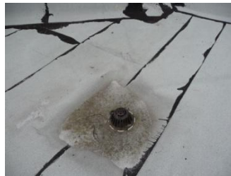
Clogged roof drains
