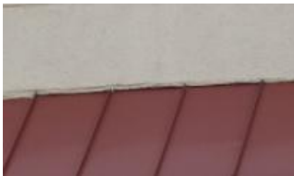
Missing / ineffective flashing
