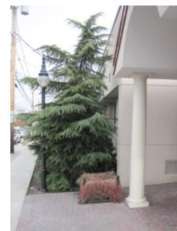
Overgrown ground vegetation touching / blocking exterior wall surfaces
