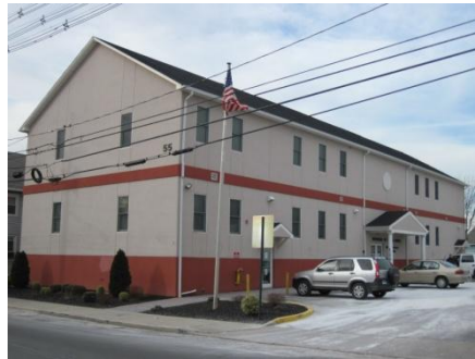
Front and Side Façade
