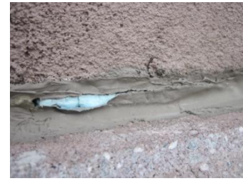
Missing/ ineffectively-applied caulk
