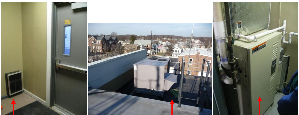
Small vestibule electric heater; typical thermostat; rooftop package unit, basement furnace & condenser
