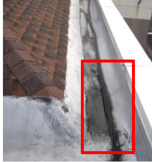
Signs of standing water/pooling
