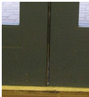
Missing/worn weather stripping
