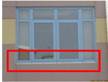
Missing window sill and drip-edge detail.
