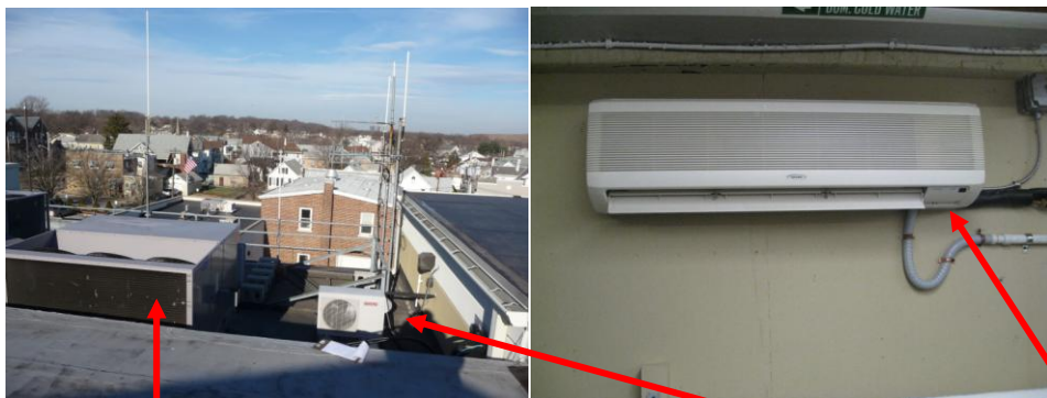
Carrier rooftop packaged unit; typical Sanyo ductless server room condenser and wall unit
