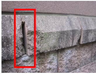
Missing/ineffectively-applied caulk/mortar
