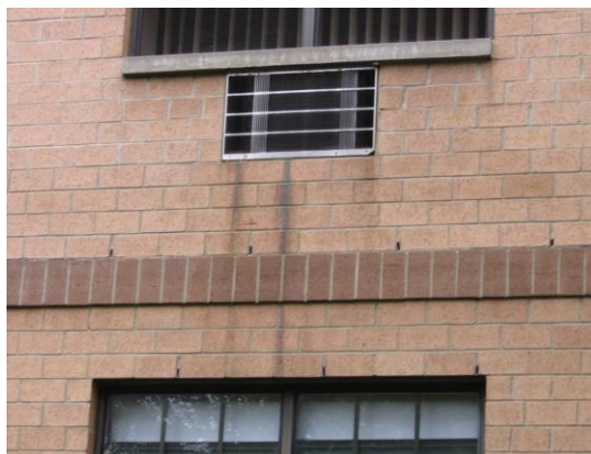
Damage to brick veneer from AC wall unit condensate
