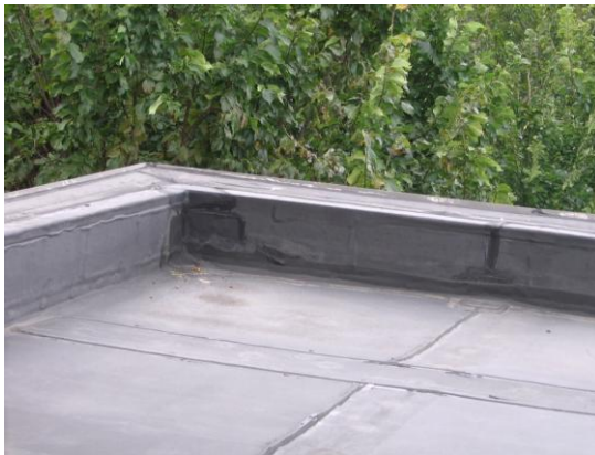
View of typical roof seams including corner
