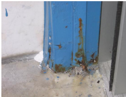
Exterior door rust build-up preventing proper seal
