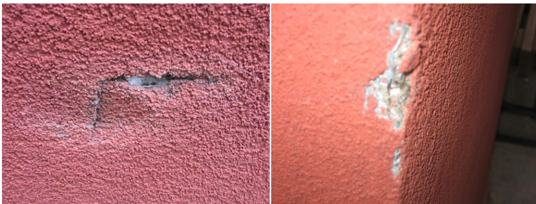
Areas showing damage to EIFS façade; leading to moisture in walls
