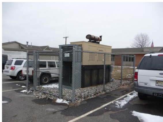
Generac 130 kW Diesel driven generator
