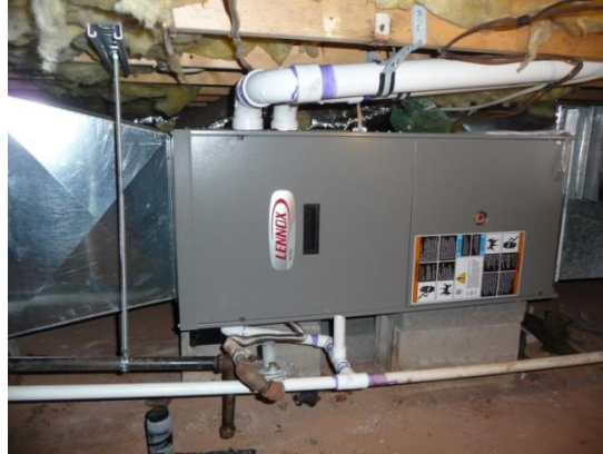
Code Enforcement condensing furnace in crawl space installed on the horizontal
