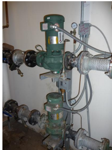
New Addition hot water circulating pumps
