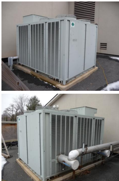
Chiller and water-glycol solution circulator pumps
