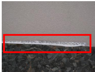
Damaged exterior wall finishes
