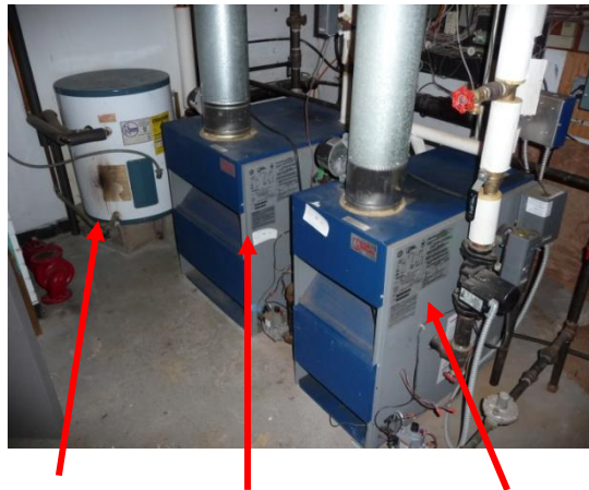
Old Courtroom area DHW; Middles section Utica boiler; Utica boiler for old Courtroom AHUs
