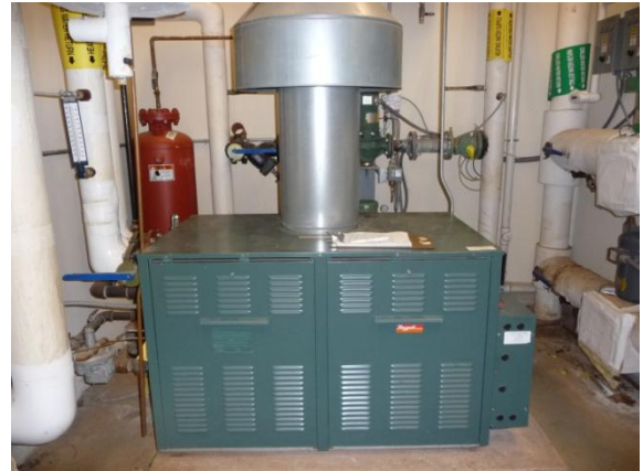
New Addition Raypack boiler
