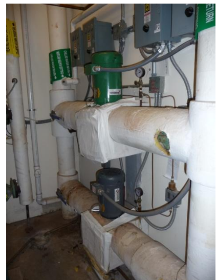
Chiller and water-glycol solution circulator pumps
