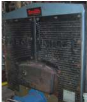
Picture: Old Cast Iron Sectional Steam Boiler at the Three Bridges School
