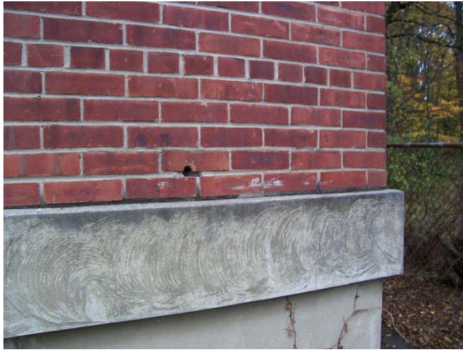
Exterior wall cracks at seams and cracked concrete blocks
