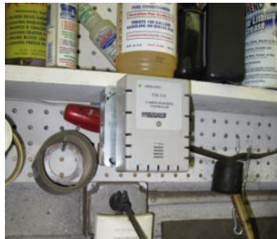
Carbon Monoxide Controller for Ventilation System
