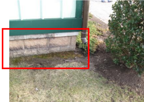
Moisture damage on exterior base and vegetation growth
