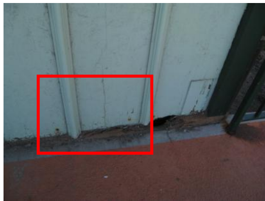
Deteriorating exterior wall finishes
