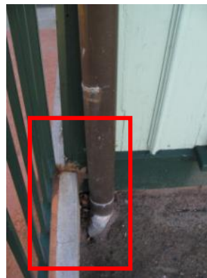
Missing downspout deflector
