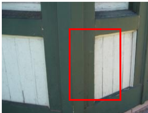
Cracked exterior wall finishes
