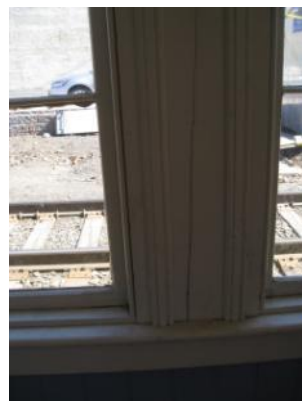
Cracked window sill on interior
