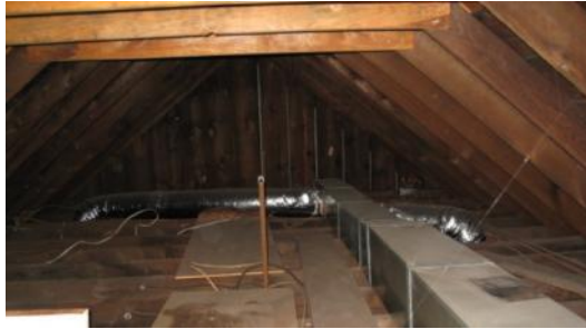
Insulated round ducts off of main air supply, leading to ceiling diffusers
