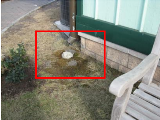
Vegetation growth at base due missing downspout deflector
