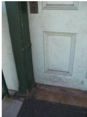
Damaged/warped door frame
