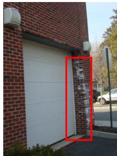
Efflorescence on brick and masonry walls indicate moisture presence within the wall cavity.
