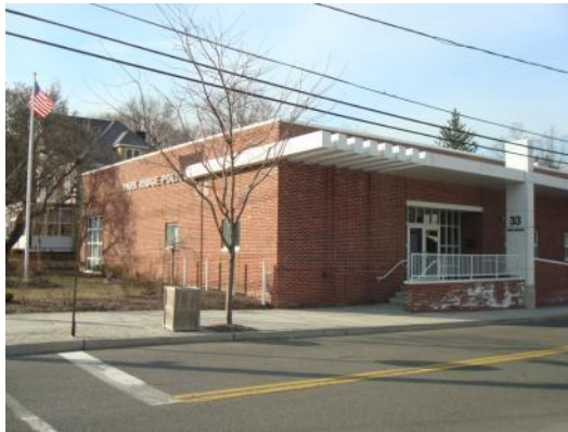
Front and Side Façade
