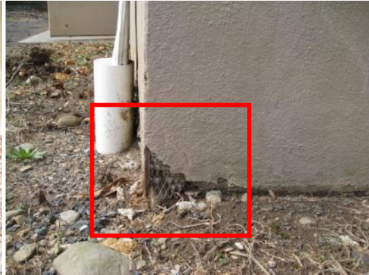
Potential water/moisture seepage through cracks detected in the slab
