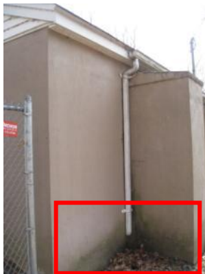
Uncontrolled roof water run-off due to missing/ineffective downspout deflector
