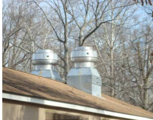
Reznor Ventilation Unit with furnace (left) and two exhaust fans on roof (right)
