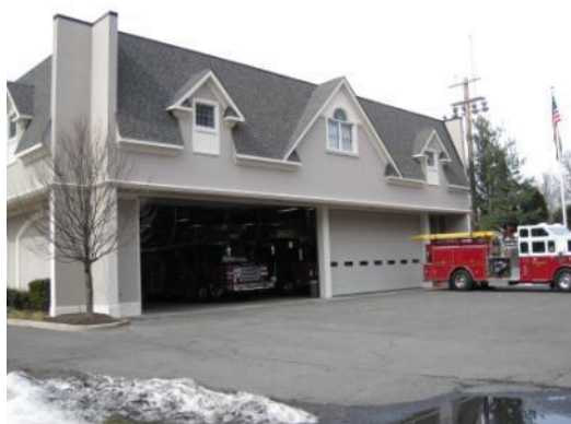
Front and Side Façade
