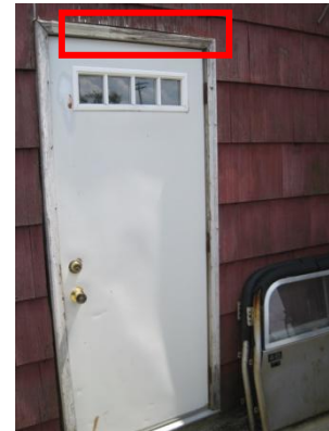
Missing/worn weather-stripping and damaged door frame
