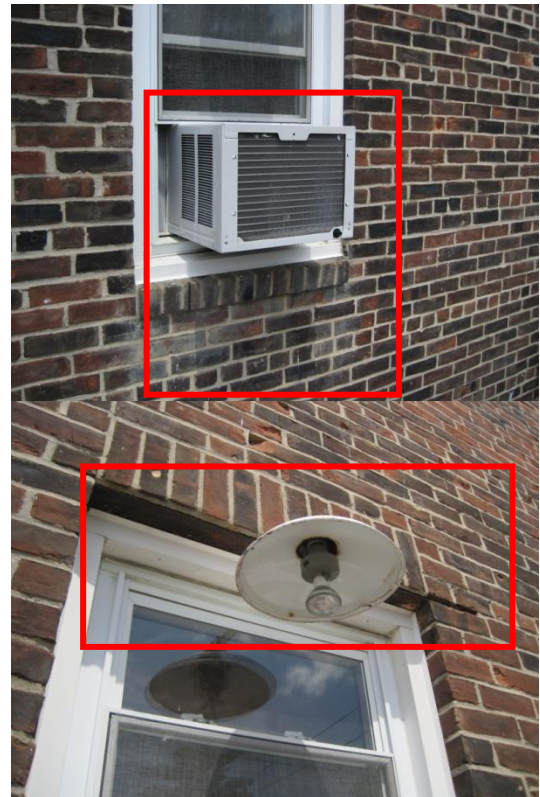
Cracked or aged caulk around frame/sill on the exterior, exterior water damage signs on areas around windows, exposed lintels creating a thermal bridge and air-leakage at sleeved window/wall air-conditioning units
