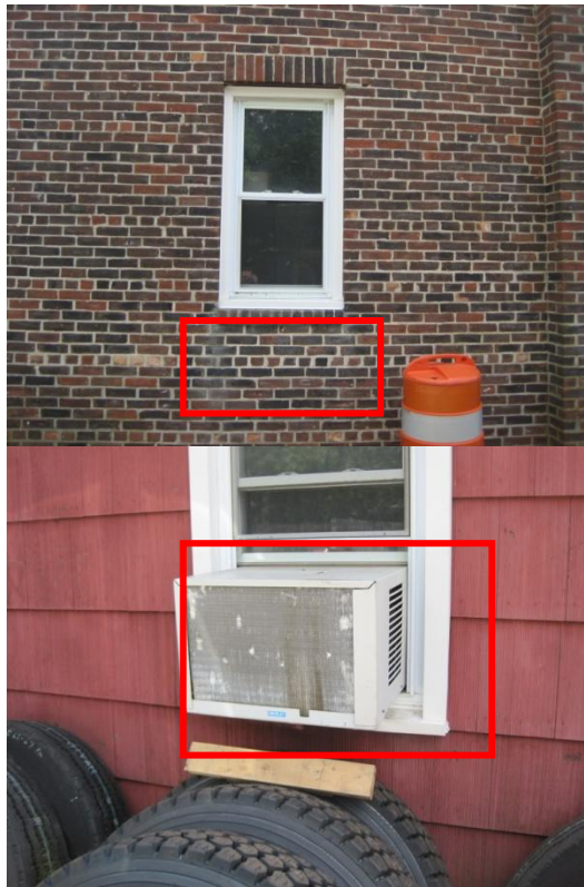
Cracked or aged caulk around frame/sill on the exterior, exterior water damage signs on areas around windows, exposed lintels creating a thermal bridge and air-leakage at sleeved window/wall air-conditioning units
