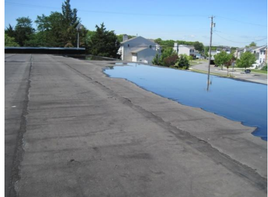
Typical Roof Surfaces. Water pooling on the flat roof
