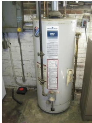
DHW heater and associated un-insulated piping
