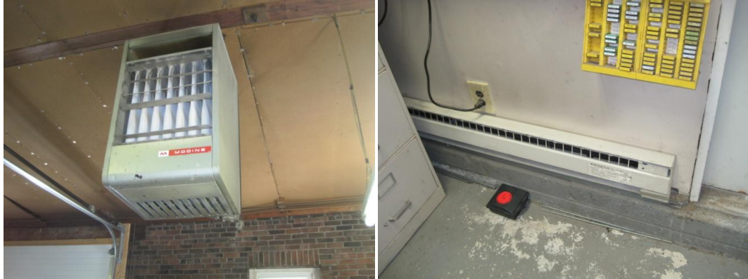
Modine gas fired heater in the Mechanics' Bay; Baseboard electric heat - Vehicle shop office
