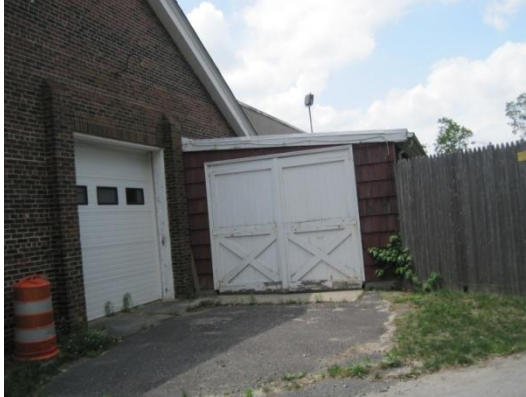
Missing/worn weather-stripping and damaged door frame
