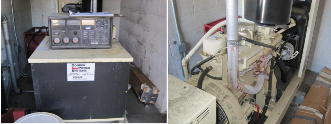
Kohler 39 kW/49 kVA emergency generator
