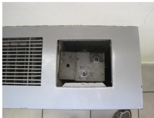
Modine cabinet heater with missing knobs for heat adjustment (typical)
