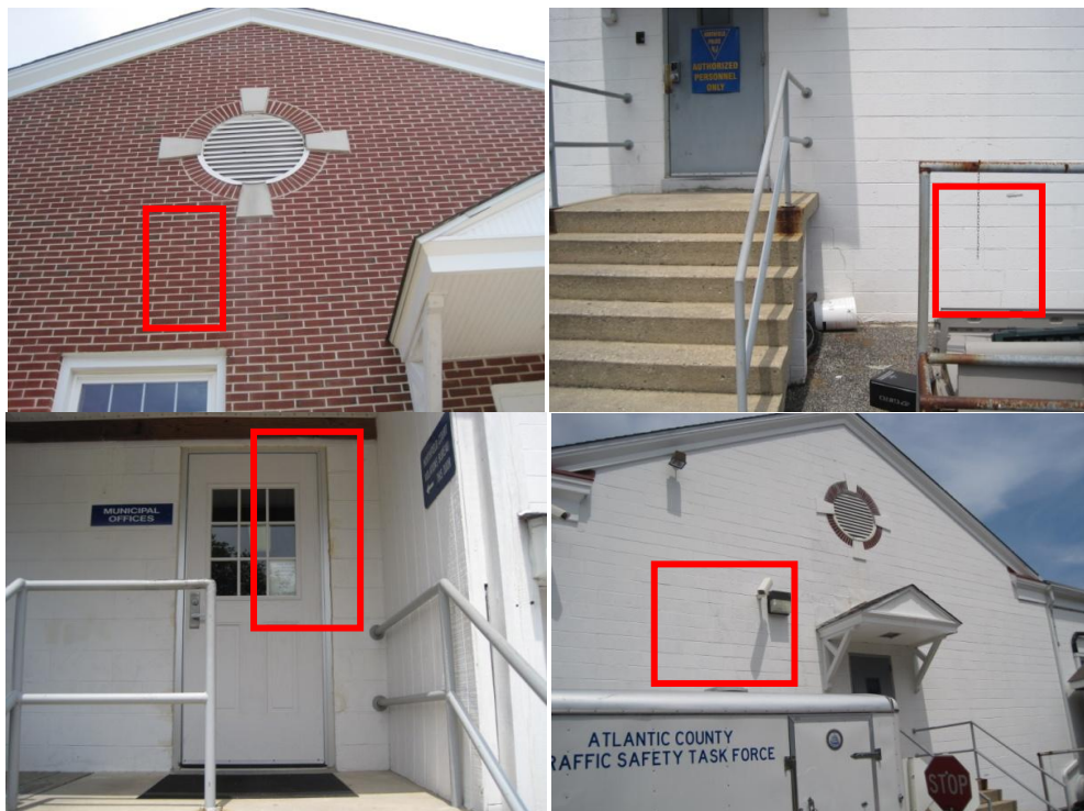
Efflorescence on brick and masonry walls indicate moisture presence within the wall cavity. Cracked/aged caulk and signs of shifted brick.
