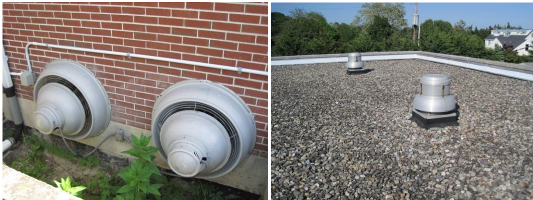
Basement exhaust fans for storage areas; Rooftop fans for Fire Dept. engine bays
