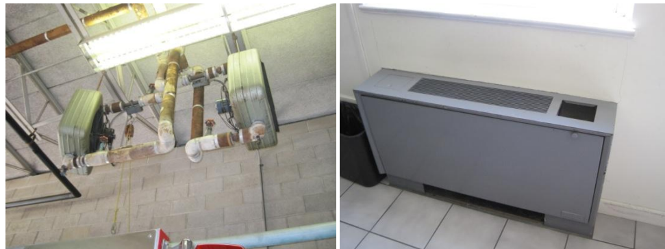
Fire Department hydronic ceiling hung units; Modine heating cabinets (typical in building)
