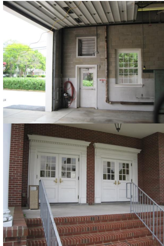
Typical exterior doors with missing/worn weather-stripping around metal doors and cracked caulk and damaged frame around some wood doors.
