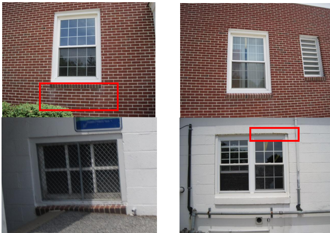
Damaged/aged window frame and air-leakage at sleeved window/wall air-conditioning units, exterior water damage signs on areas around windows
