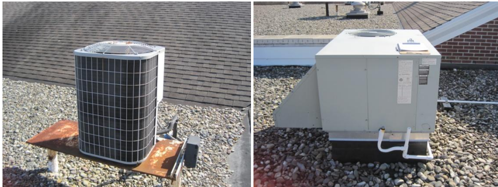
Police Department rooftop heat pump condenser; Fire Department rooftop packaged AC
