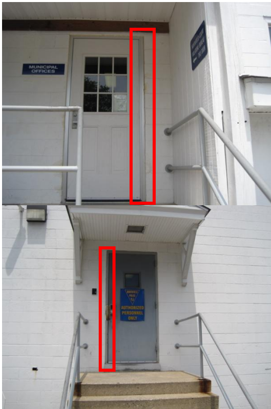
Typical exterior doors with missing/worn weather-stripping around metal doors and cracked caulk and damaged frame around some wood doors.
