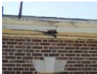
Deteriorating roof trim and compromised roof flashing detected
