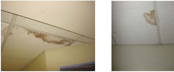
Signs of mold/water damage on interior finishes
