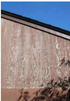
Sun damaged exterior wall finishes
