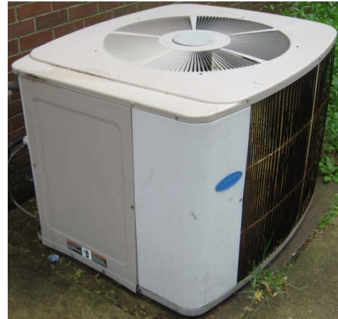
Figure 2: Carrier condensing unit
