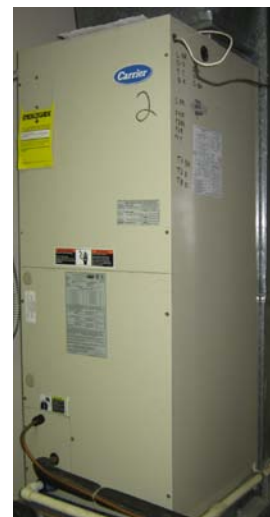
Figure 1: Carrier forced-air furnace
