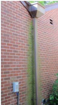
Uncontrolled roof water run-off due to defective or clogged gutters and downspouts
