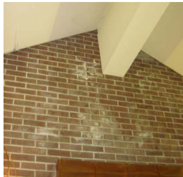
Efflorescence on interior brick walls indicate moisture presence within the wall cavity.
