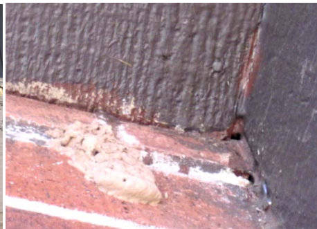
Damaged exterior wood trim caused by different types of insects, according to building maintenance personnel.
