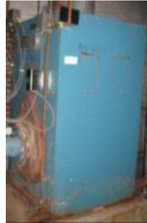
Figure 1: Burnham steam boiler
