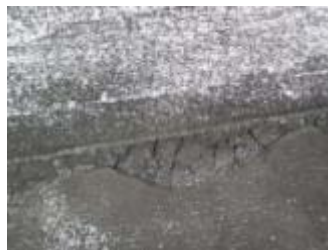
Deteriorating roof membrane and patches
