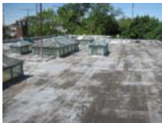
The roofing material has reached the end of its useful lifespan.
