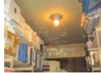
Signs of moisture damage on interior finishes
