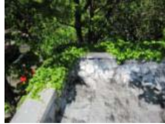
Ground vegetation touching/overhanging roof surfaces
