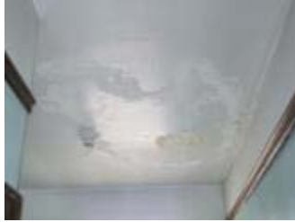
Signs of water damage on interior finishes
