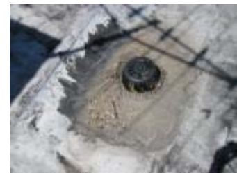
Clogged and damaged roof drains
