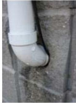
Un-caulked/un-sealed exterior wall penetrations
