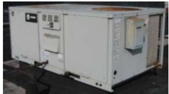
Figure 2: Trane packaged DX rooftop unit
