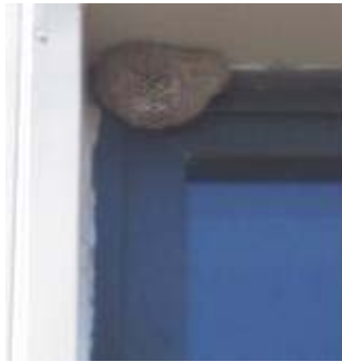
Insect nesting in exterior wall cracks and cavities
