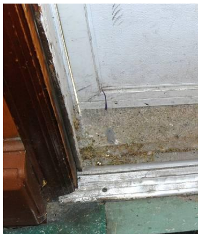
Missing or Worn Weather-Stripping at front door
