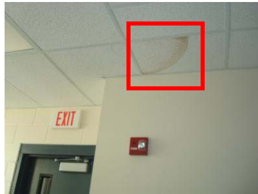
Soffit paint peeling; wet ceiling tile - most likely from a roof leak
