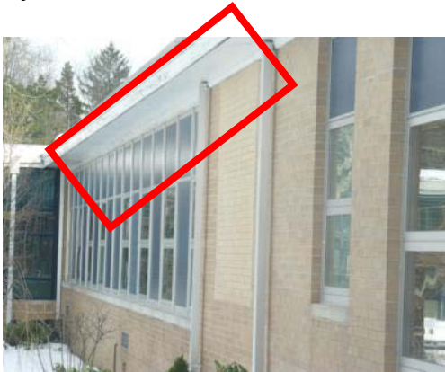
Soffit paint peeling; wet ceiling tile - most likely from a roof leak
