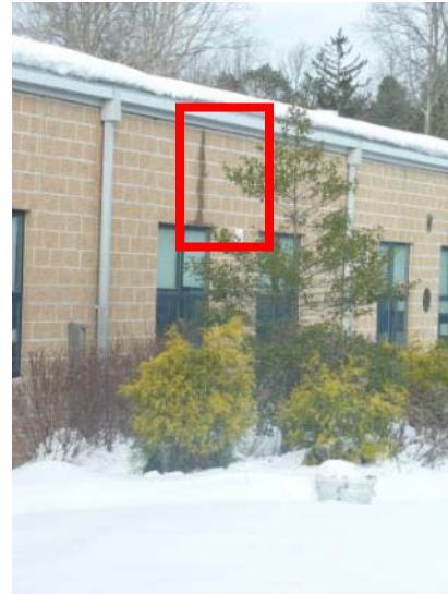
Exterior walls show signs of water leakage from roof and flashing compromising wall insulation
