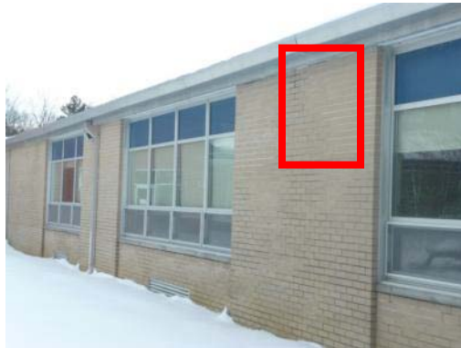
Exterior walls show signs of water leakage from roof and flashing compromising wall insulation
