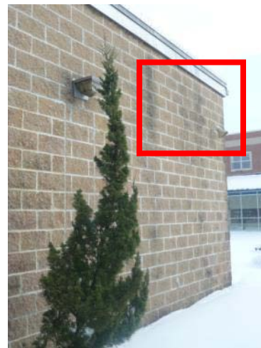
Exterior walls show signs of water leakage from roof and flashing compromising wall insulation
