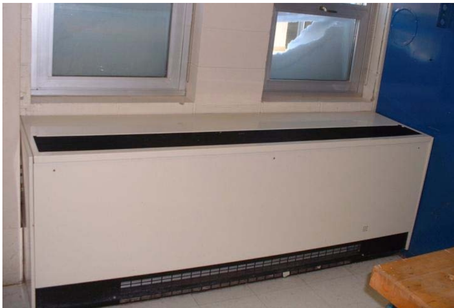
Typical classroom unit ventilator, providing outside air ventilation, heating and cooling
