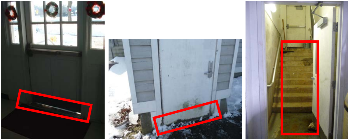
Front door in need of stripping (left), Back basement door deteriorating (center), Water on basement stairs (right)
