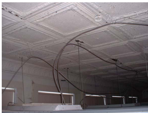
Old metal ceiling above the drop ceiling
