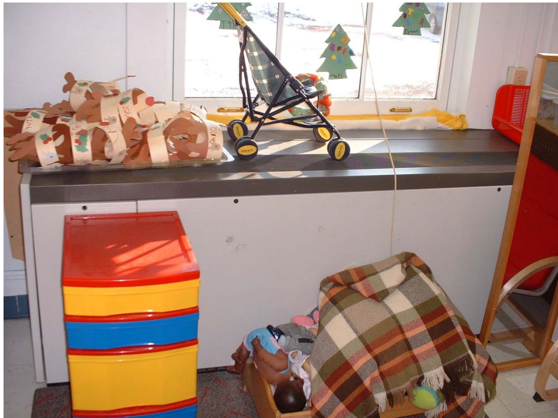
Typical classroom unit ventilator, providing outside air ventilation and cooling
