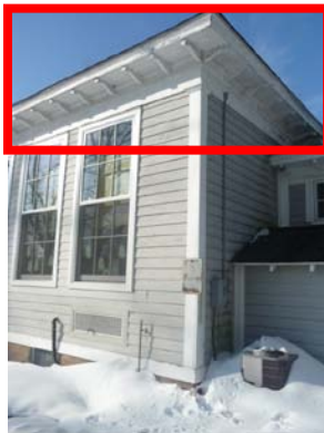
Soffits in need of gutters
