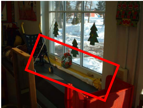
Window latching issues have caused occupants to use towels to seal bottom of windows
