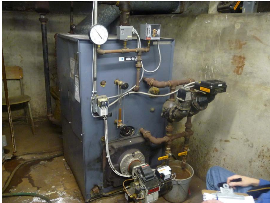
Weil McLain steam boiler in basement mechanical room
