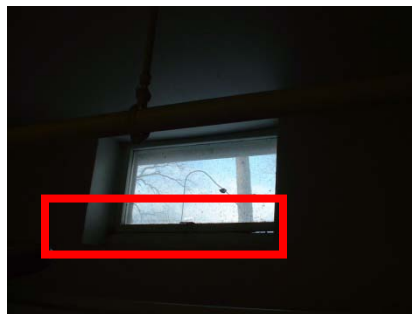
Basement window in need of perimeter sealing and caulking
