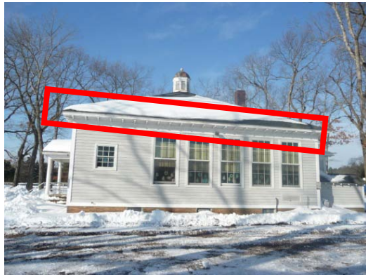
Soffits in need of gutters
