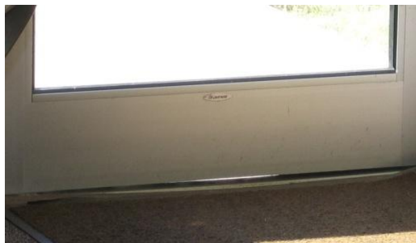
Doors not closing completely and missing weather stripping
