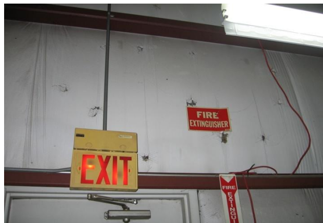
Damaged fiberglass insulation blankets
