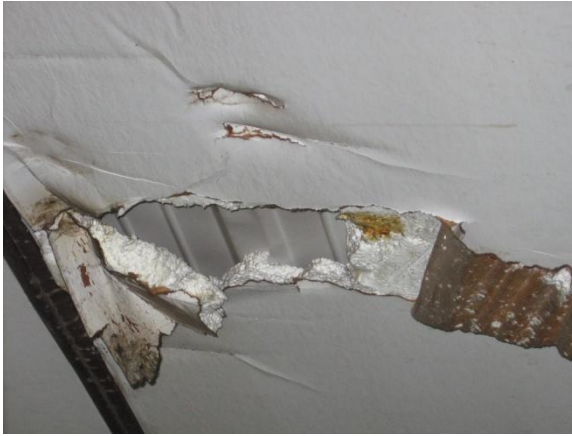
Some roof insulation boards were found to be damaged
