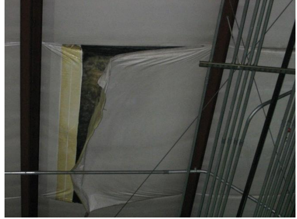
Some roof insulation boards were found to be damaged
