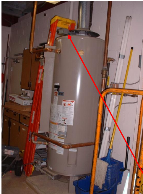
Domestic Hot Water heater with automated closing flue gas damper
