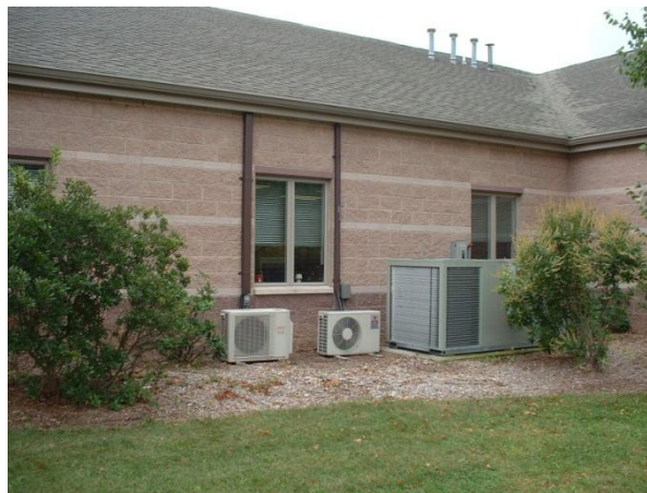
Two small server room condensing units next to a corner building space condenser
