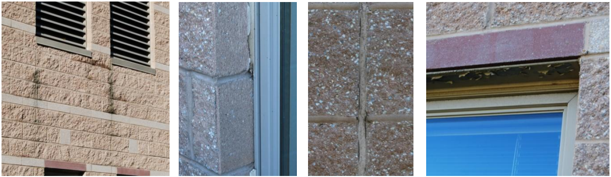
Caulk and mortar issues
