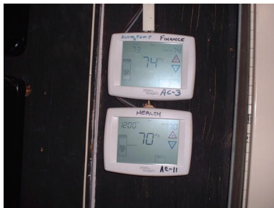
New independent temperature controls migrated away from the BMS system
