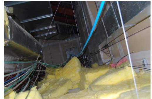
Unevenly distributed or missing 10" fiberglass batt insulation on top of ceiling tiles
