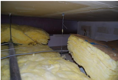
Unevenly distributed or missing 10" fiberglass batt insulation on top of ceiling tiles
